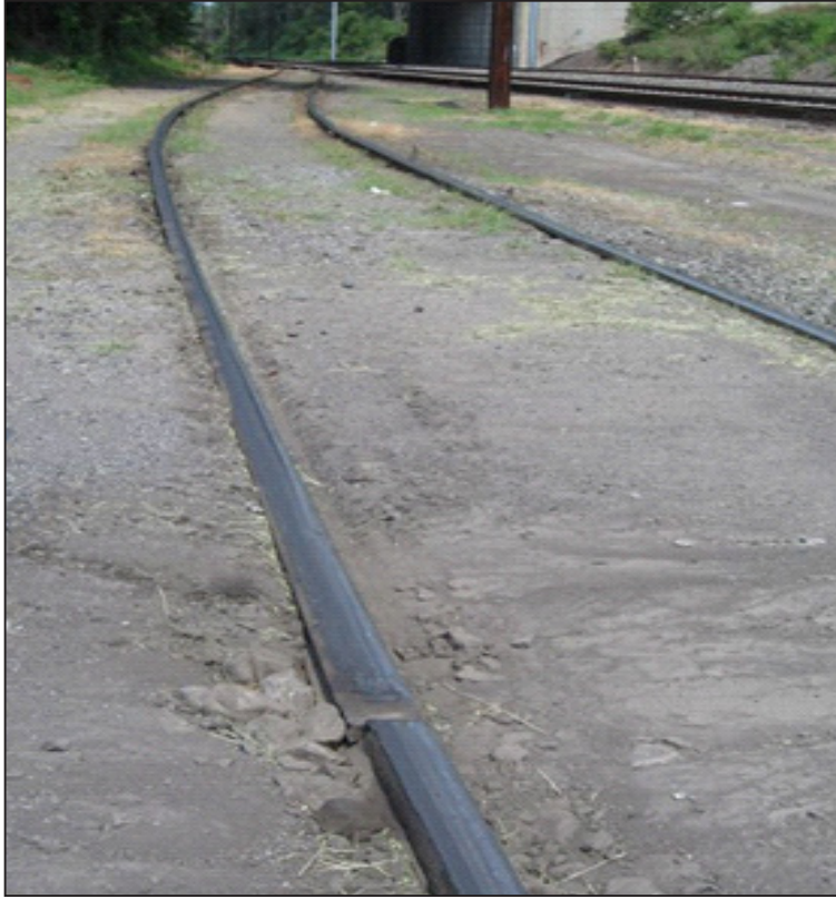
Before: Rails are warped, cracked and worn at several spots along the main line, increasing the risk of derailment and forcing traffic to move slowly over unstable areas of rail.
